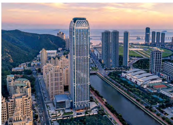
The 216-room Pan Pacific Dalian is strategically located on Youting Road, with breathtaking views of the Yellow Sea and surrounding hills.
