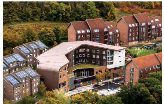
Varley Park, a complex of student residential halls in Brighton, United Kingdom, comprising 771 operational beds.
